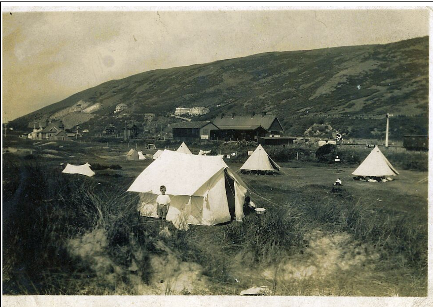
Above— 1937 -Colin's elder brother outside the family tent, just behind the tents is Aberdovey Railway Station that made it all possible I suppose.
